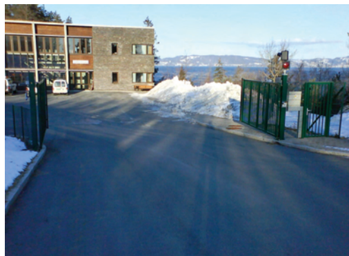
Figure 1. Høvringen wastewater treatment plant is situated 2 km north west of the city near Trondheim fjord.
