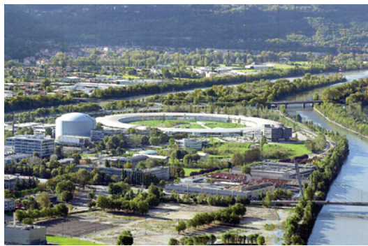
An view of ILL. The neutron reactor is seen as the white cylinder to the left in the picture. With courtesy of the ILL.
