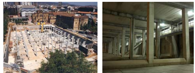
Fig. 4. Detention tank construction (left). Detention tank inside (right)
