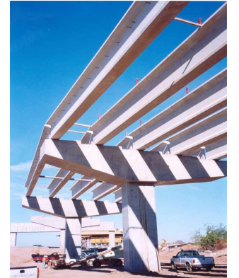
Figure 2. General view of the construction of vehicle lanes [1]
