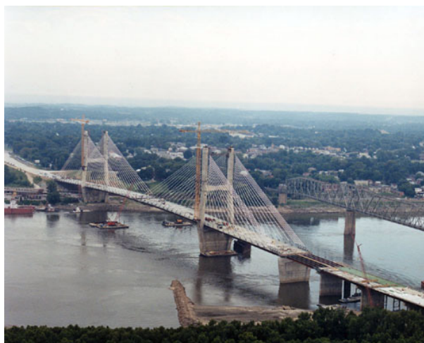
Figure 1. Construction of the Bill Emerson Memorial Bridge Source: http://www.modot.state.mo.us/local/d10/emersonbridge
