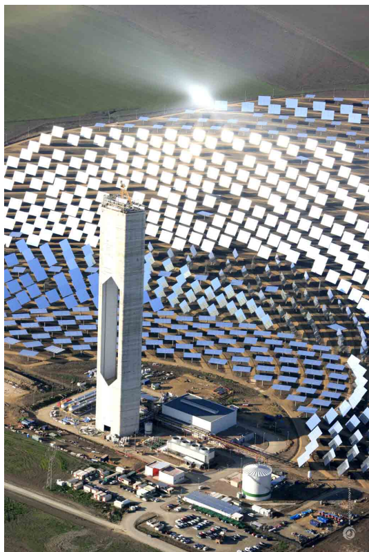
Fig. 1. Abengoa PS20: a 20Mw solar power tower
