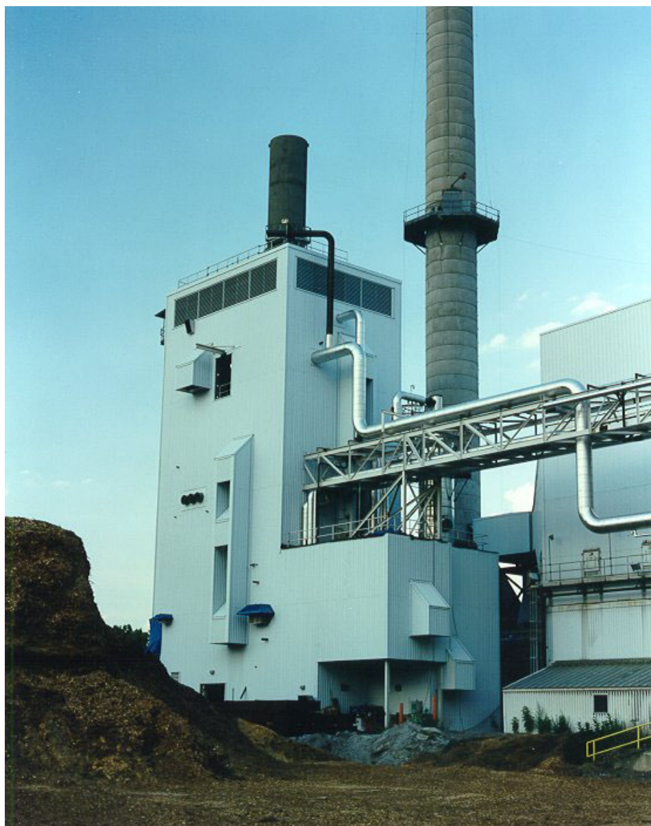
Figure 2 SilvaGas 400 Dry Ton per Day Commercial Scale Facility
