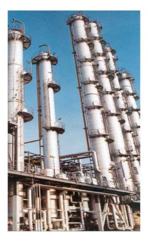
Fig. 12: Main packed columns for BASF NMP butadiene process /8/
