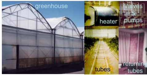
(a) Greenhouse heated by aerial pipes
