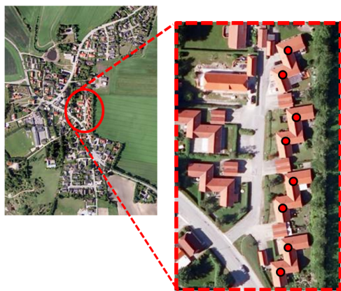
Fig. 2. The demonstration site including 8 residential houses with photovoltaic cells on top of the roofs
