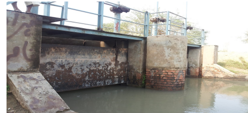
Fig. 6. Upstream Gate at Khaira Distributory.
